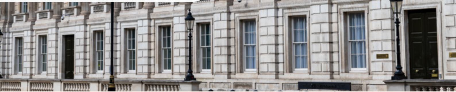
The Cabinet Office
